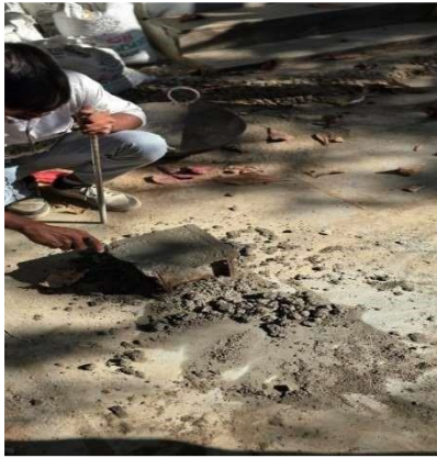
Casting Cube moulds
