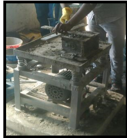
Fig:8. Compaction by vibrator
