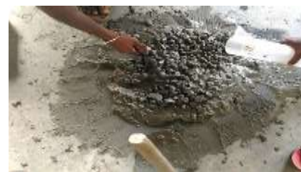
Mixing the concrete
