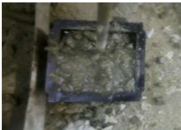
Preparation of Concrete cube
