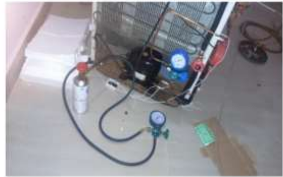
Fig 3.5.1 Charging of Refrigerant R600a
