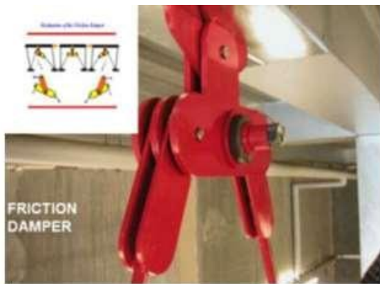
Using rotational friction dampers in retrofiting
