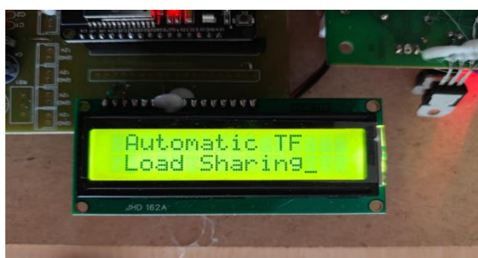
Fig.3: LCD display indicating automatic transformer load sharing operation
