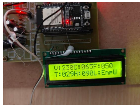
Fig. 3: LCD display showing real-time substation operating parameters
