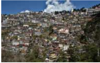
Figure 1: Buildings on sloping ground
