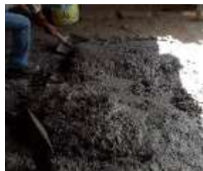
Fig 5: Mixing of concrete
