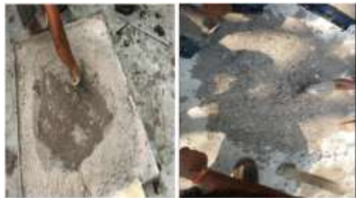
Mixing of Geopolymer concrete
