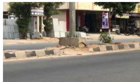
Figure 4.6 At chainage 3.000 Km,
