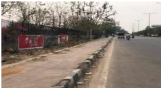
Figure 4.1: At chainage 0.800km,
